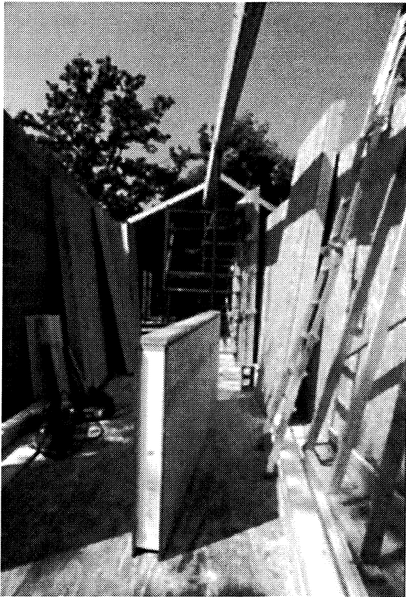
Fig. 2 Photo describing the use of modular materials that determined the length, width and breadth of the house as it fit into the narrow site conditions. Structurally insulated panels were used to test and confirm the added benefits of thermal control of this product. The SIS used materials that offered an option to traditional, stick built construction methods.
