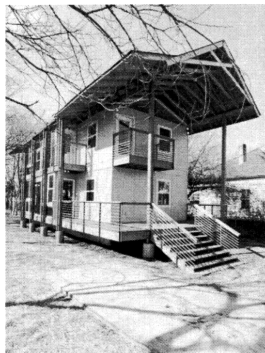
Fig. 5 This photo illustrates the use of a front porch to create an exterior room that also aids in the control of interior temperature. It also had an oversized stair platform and created a place for gathering and participating with the street and community. The addition of a porch was intended to be an economical use of space. House 2 used a back porch intended for exterior dining.
